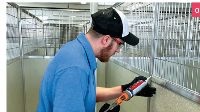
01 Kennels units are properly sealed to protect the longevity and safety of kennel materials.
