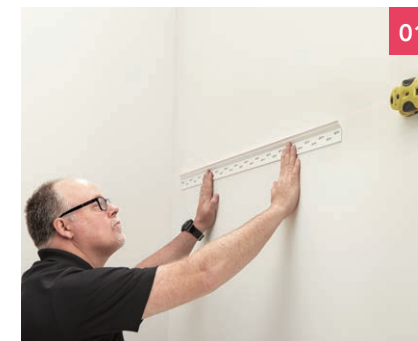
01 Field measurements are confirmed to ensure seamless installation.
